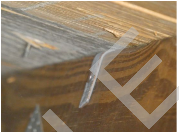
ROOF TO WALL ATTACHMENT
