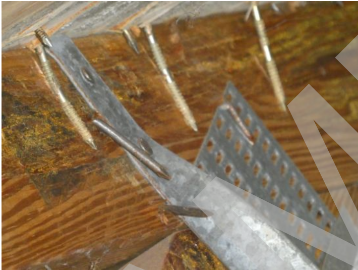
ROOF TO WALL ATTACHMENT
